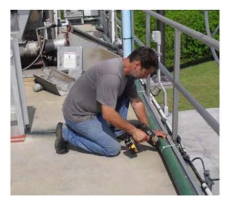
Secure hose with zipties and drill 30- 1/4"diameter holes evenly spaced facing the odor source. Up to a maximum of 300 feet.
